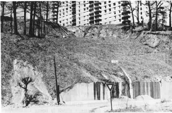
Figure 9. Debris slide underlain by Fort Payne Formation located at EMIN 4 (north end of Cameron Hill).
