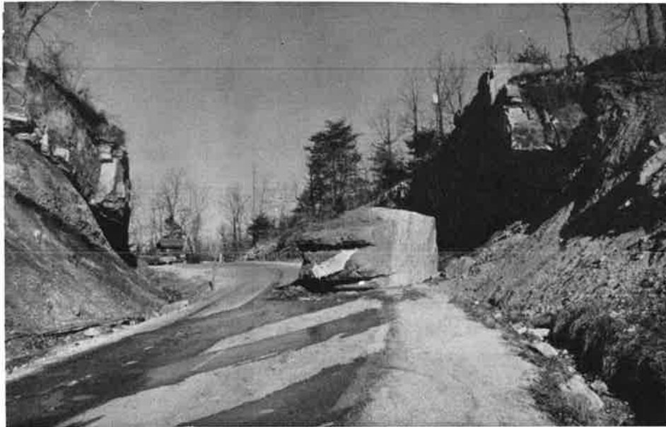
Figure 20. Rockfall in Gizzard Group caused by undercutting of massive sandstone by rapidly weathering shale, located at EMIN 3 (top of Elder Mountain Road).
