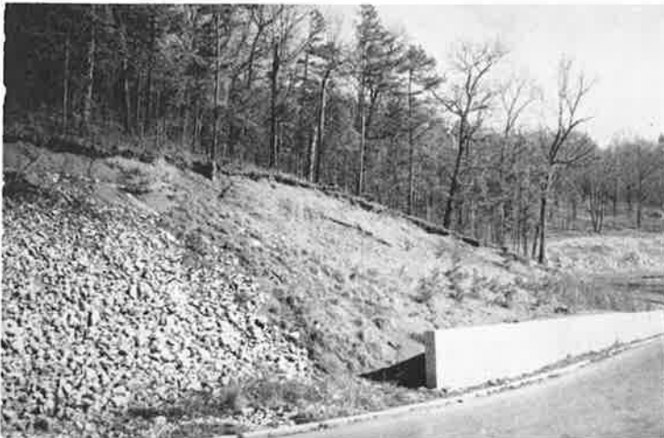
Figure 16. Large slump in Chickamauga Group colluvium and residuum located at EMIN 7 (to rear of City View Apartments, east side of Glenwood Drive).
