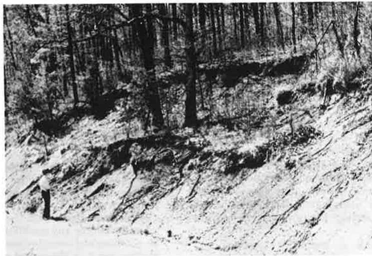
Figure 3. Typical roadside slump in colluvium overlying the Pennington Formation.
