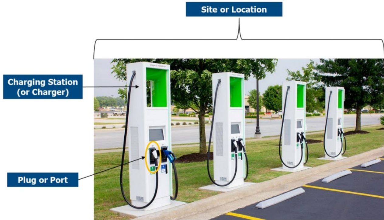
Figure 1. Example Fast Charging Site and Terminology
