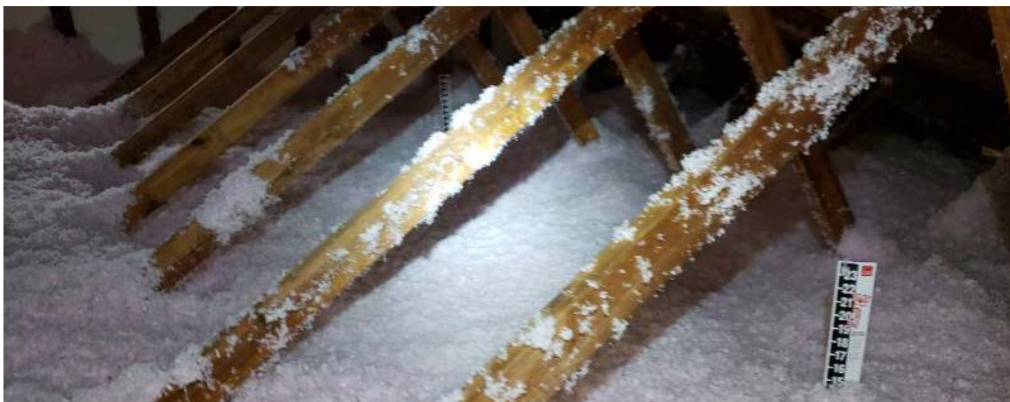
Home Uplift home's attic after the addition of insulation.
