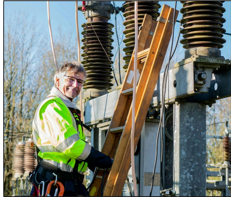
Worker at electrical transformer substation by Rene Terp
