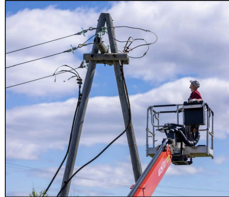
Worker repairing power lines by Sergei Serostin
