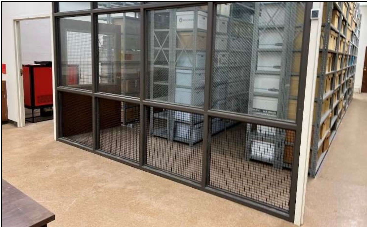
Pinson repository renovations – note the dehumidifier frame left and grates in the glass wall and doors between the lab and repository to improve air flow throughout the facility.
