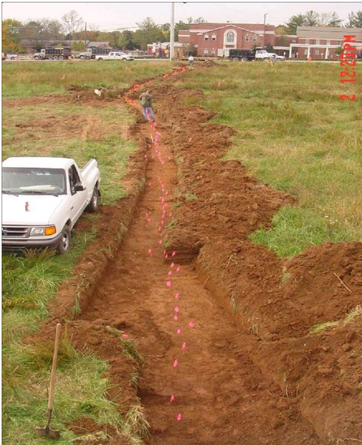
Figure 66. View west of the outer palisade (Feature 20) relative to the local topography. Project construction on Hillsboro Road underway in background.
