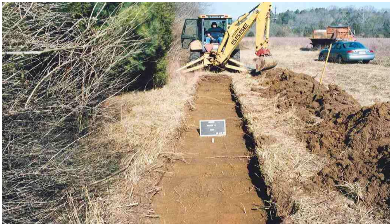
Figure 13. View north of Trench E showing the shallow depth of subsoil in the northhalf of the project ROW.
