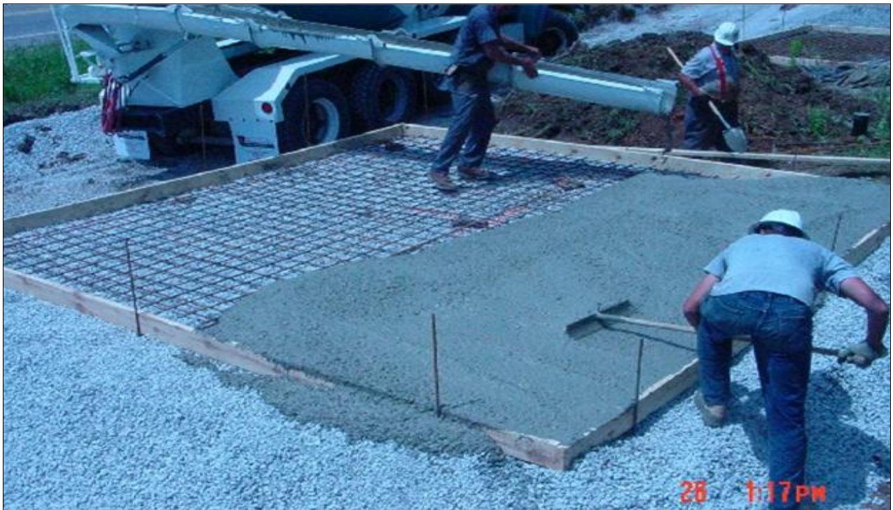
Figure 4. Concrete being poured into a rebar reinforced form covering a burial at Kellytown.
