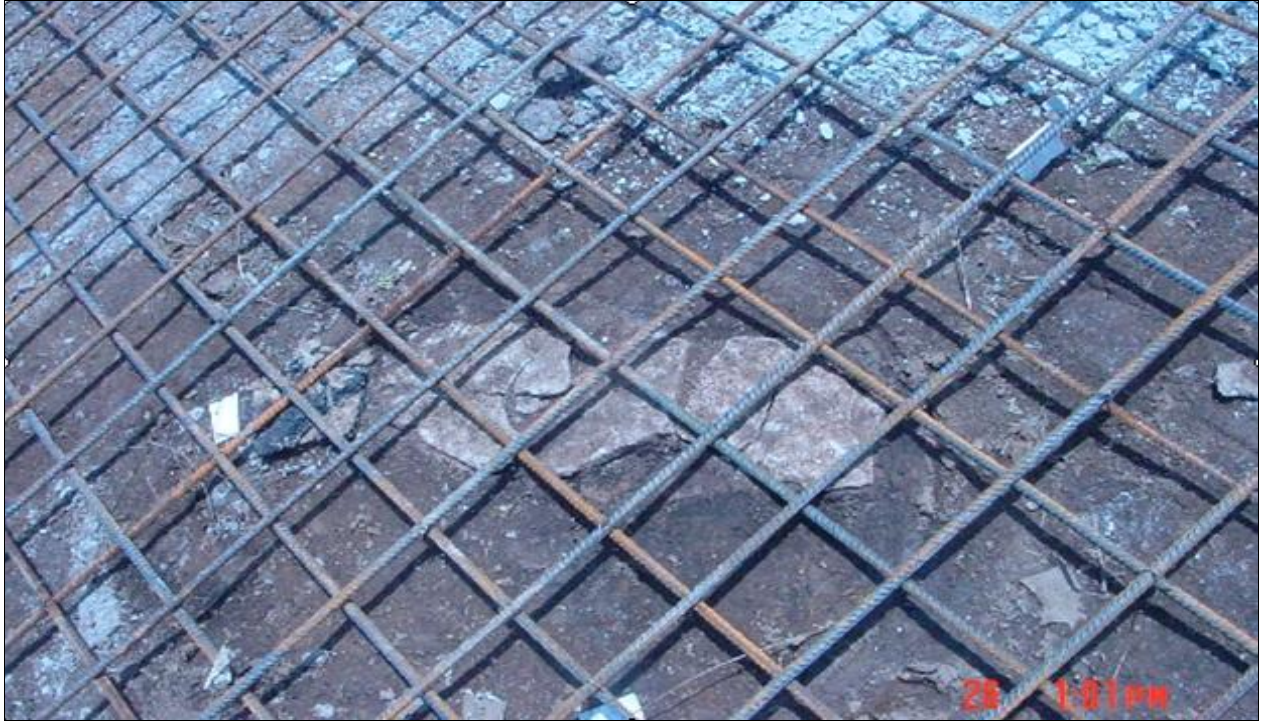
Figure 3. Rebar reinforcement in wooden form placed over a child stone box grave at Kellytown.
