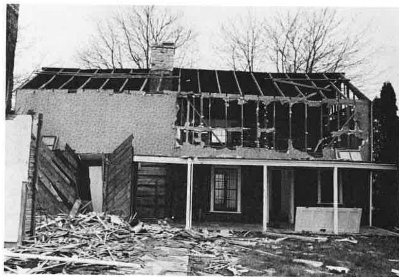
FIGURE 5. South elevation, west pen pièce sur pièce , east pen "V" notch, Knox County, Tennessee.
