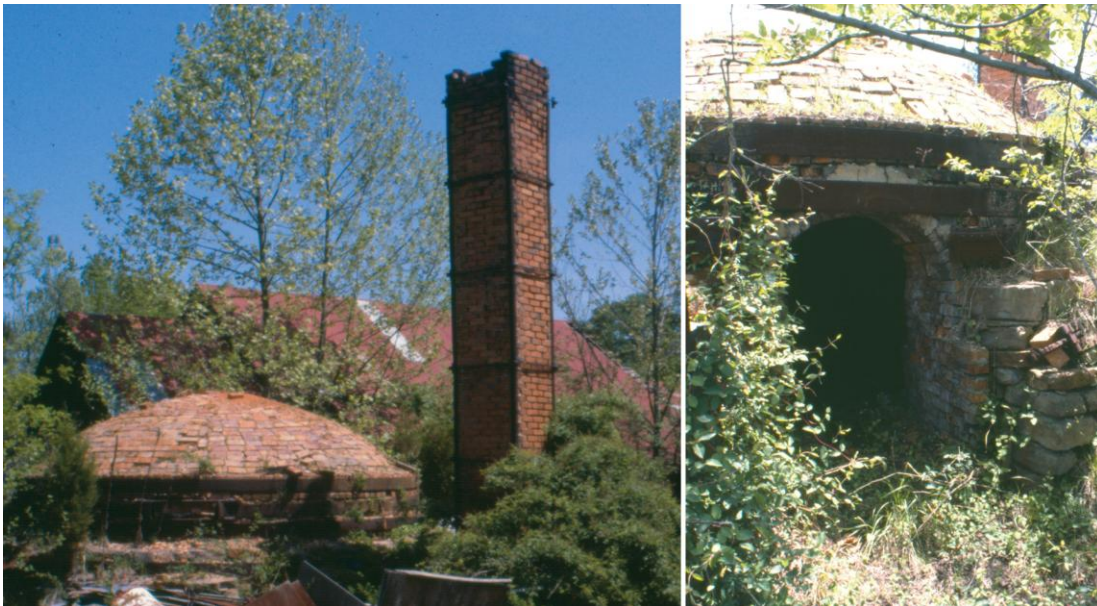
Figure 1-9. General view and close-up of the loading door of a downdraft kiln once used by the Waco Pottery in Waco, Kentucky (from slides taken in 1981).
