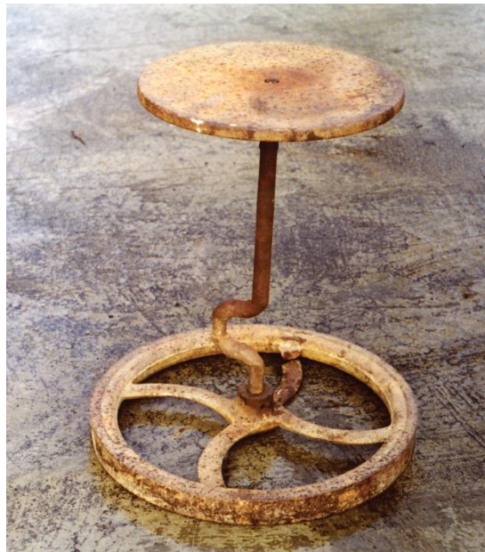
Figure 2-35. Metal portion of a potter’s treadle wheel (minus the wooden frame and other parts) that was retained by Sam McFarland after closing of the M. P. Harmon pottery (it belongs to a descendant of Sam McFarland).
