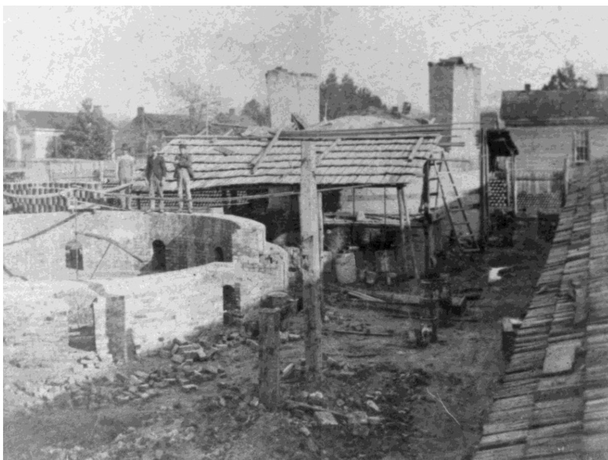
Figure 2-260. Photograph showing kiln construction in the backyard of the Pinson Pottery (courtesy of Sybil K. Thornton).
