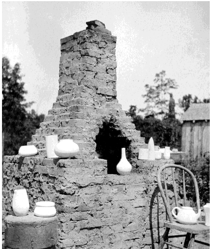
Figure 2-272. A kiln at the Nonconnah pottery with pottery wares waiting to be fired (courtesy of J. Thomas Case and Rodney H. Leftwich).
