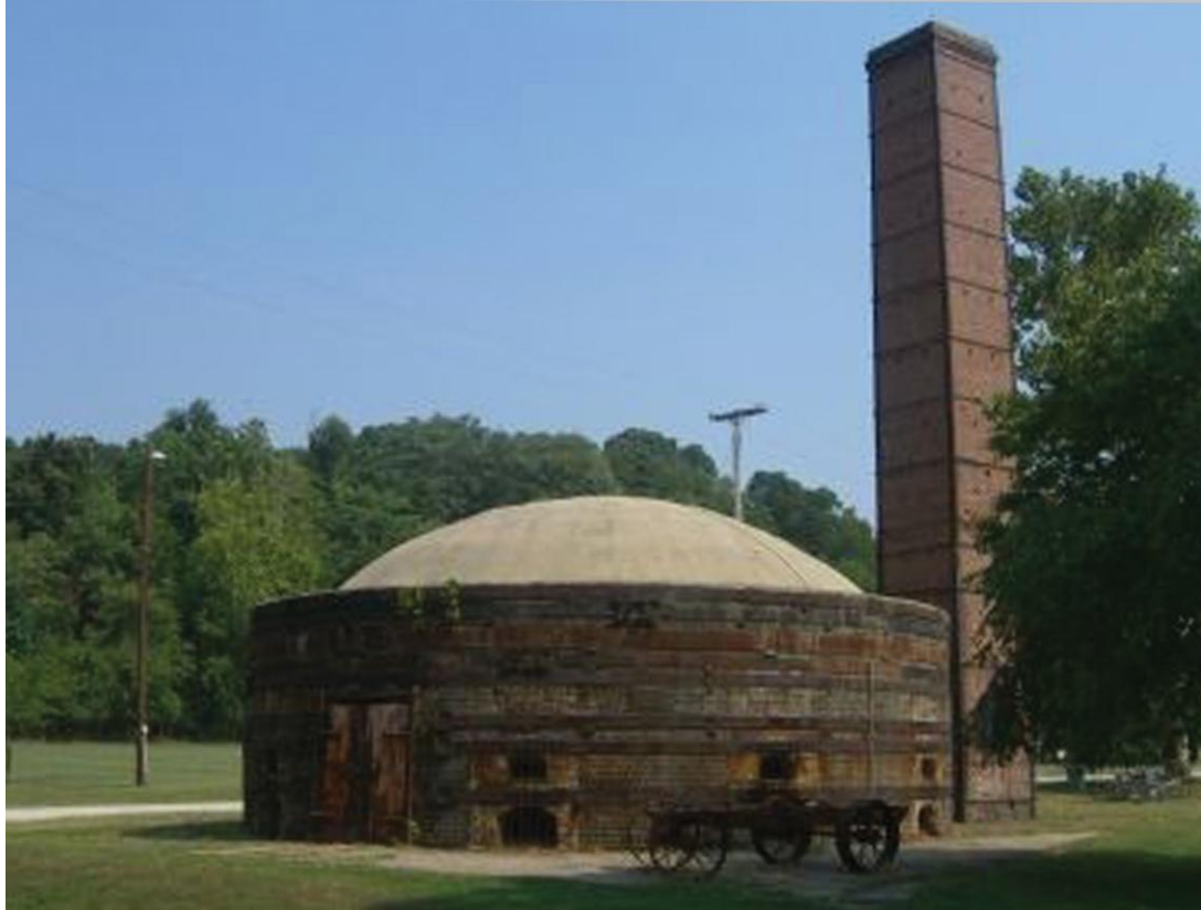
Figure 1-8. A downdraft “beehive” brick kiln preserved in a Fairfax County, Virginia park (photograph courtesy of Kevin White, The Historical Marker Database <HMdb.org>).
