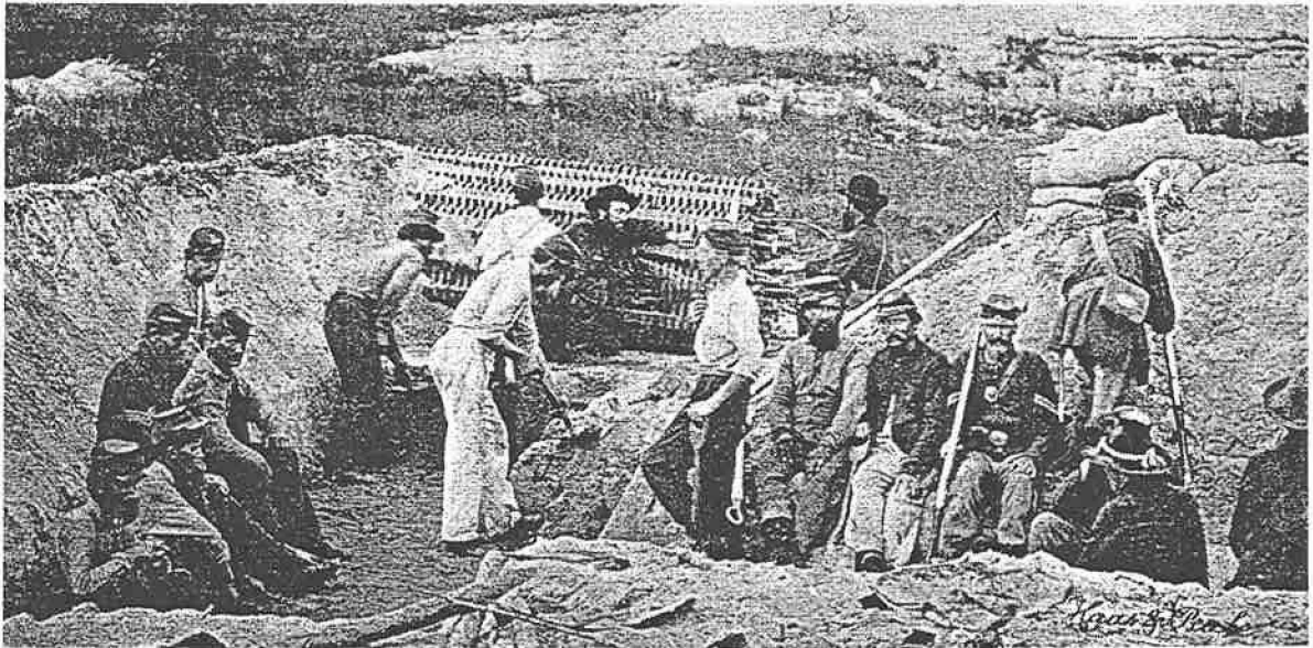
Federal soldiers digging a sap using a sap roller (from a National Archives photograph)
