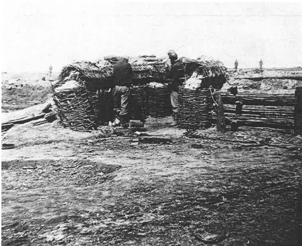
Figure 12. Earthworks constructed using gabions (United States Army Military History Institute [USAMHI]).
