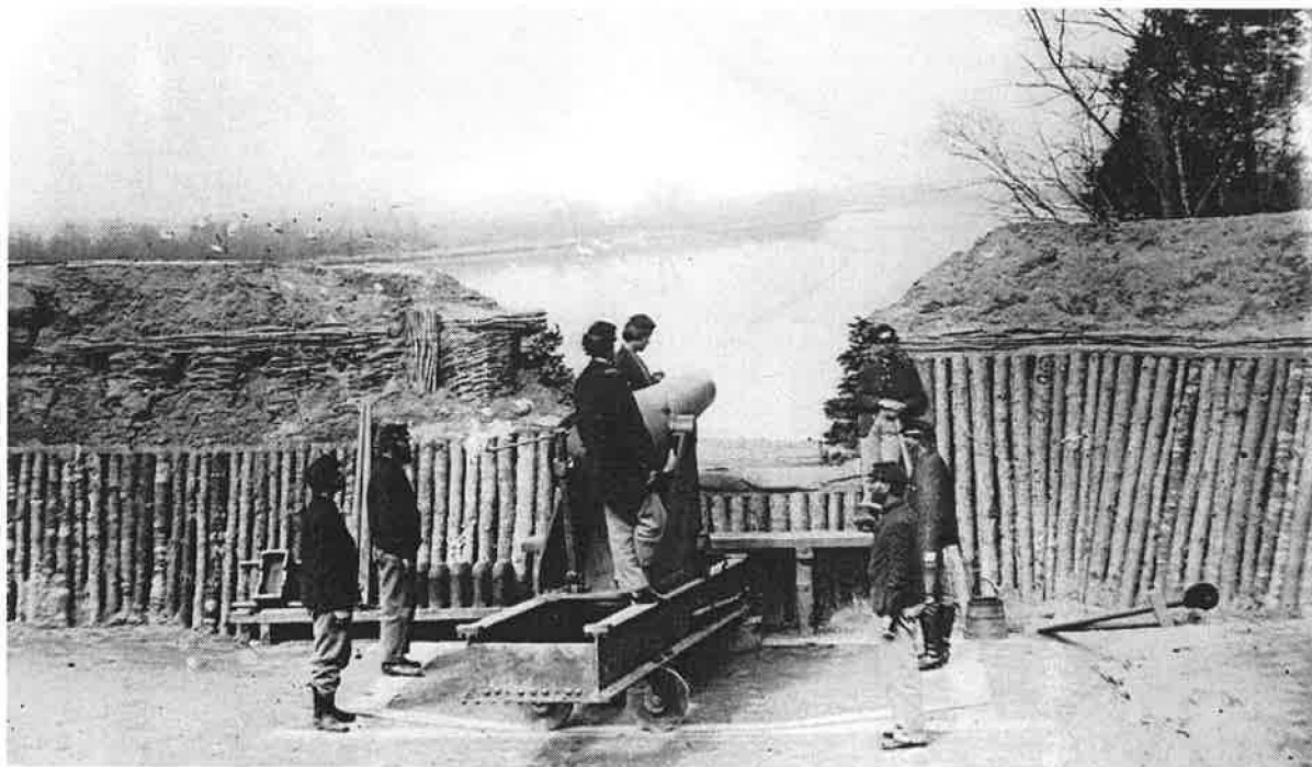
Figure 13. Earthworks of composite construction used in a river battery at Chattanooga (TSL & A, Image 147).
