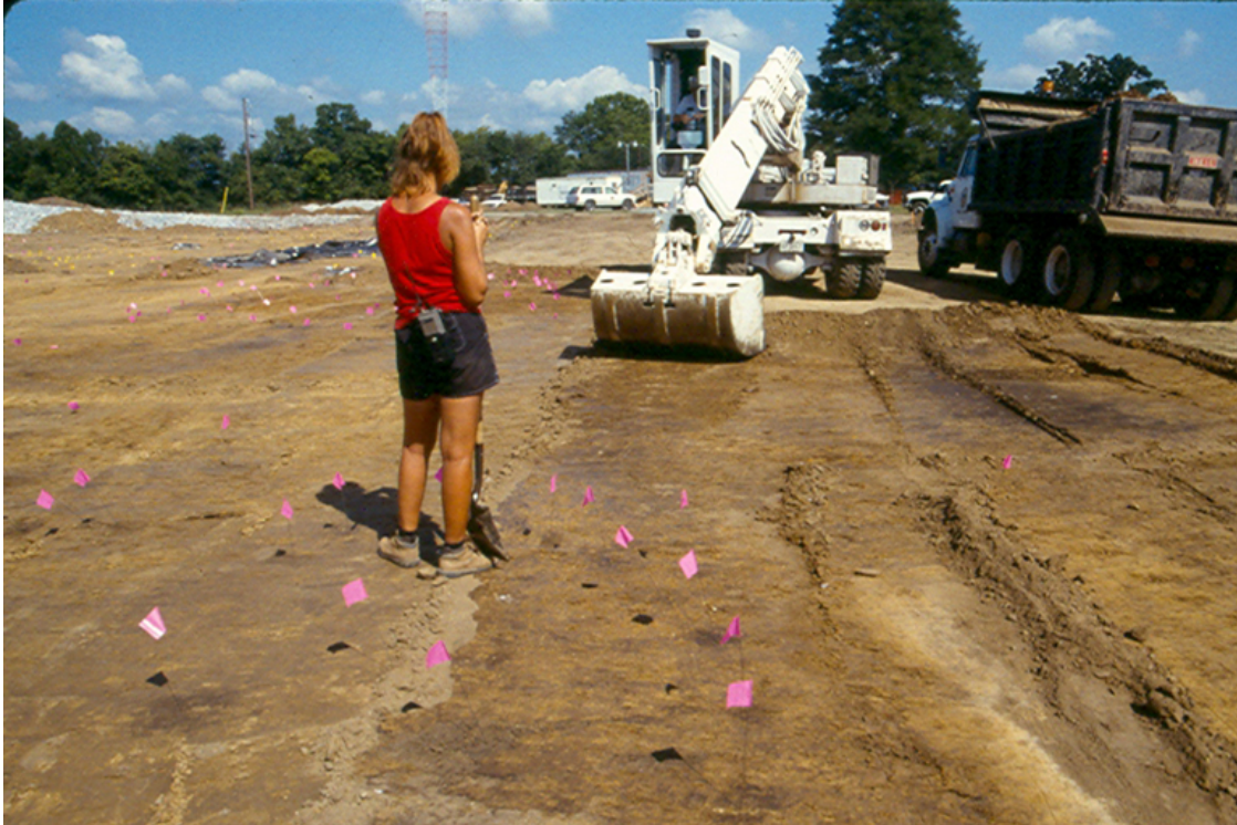
Figure 9. Stripping operations in parking lot area, looking north.
