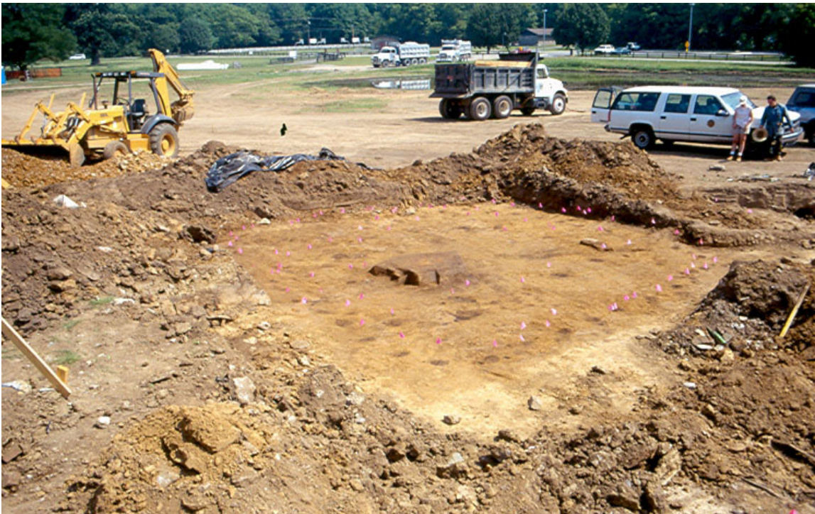
Figure 25. Structure 3 exposed in field, looking northeast.
