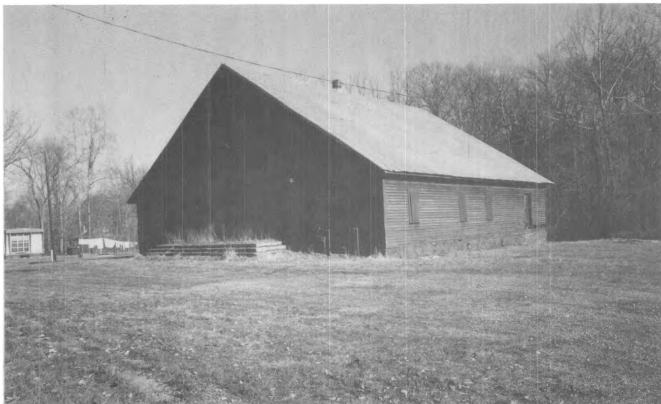
Figure 31. Cumberland Furnace Commissary (Dickson County 324).
