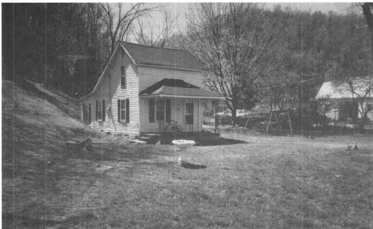
Figure 45. Rockdale Row House Number 5 (Maury County 427).
