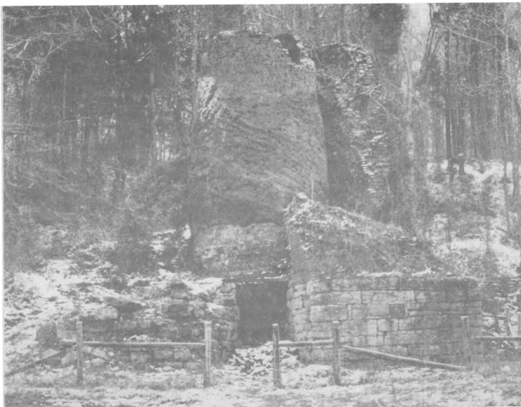
Figure 16. Remains of Brownsport (II) Furnace (40DR86).
