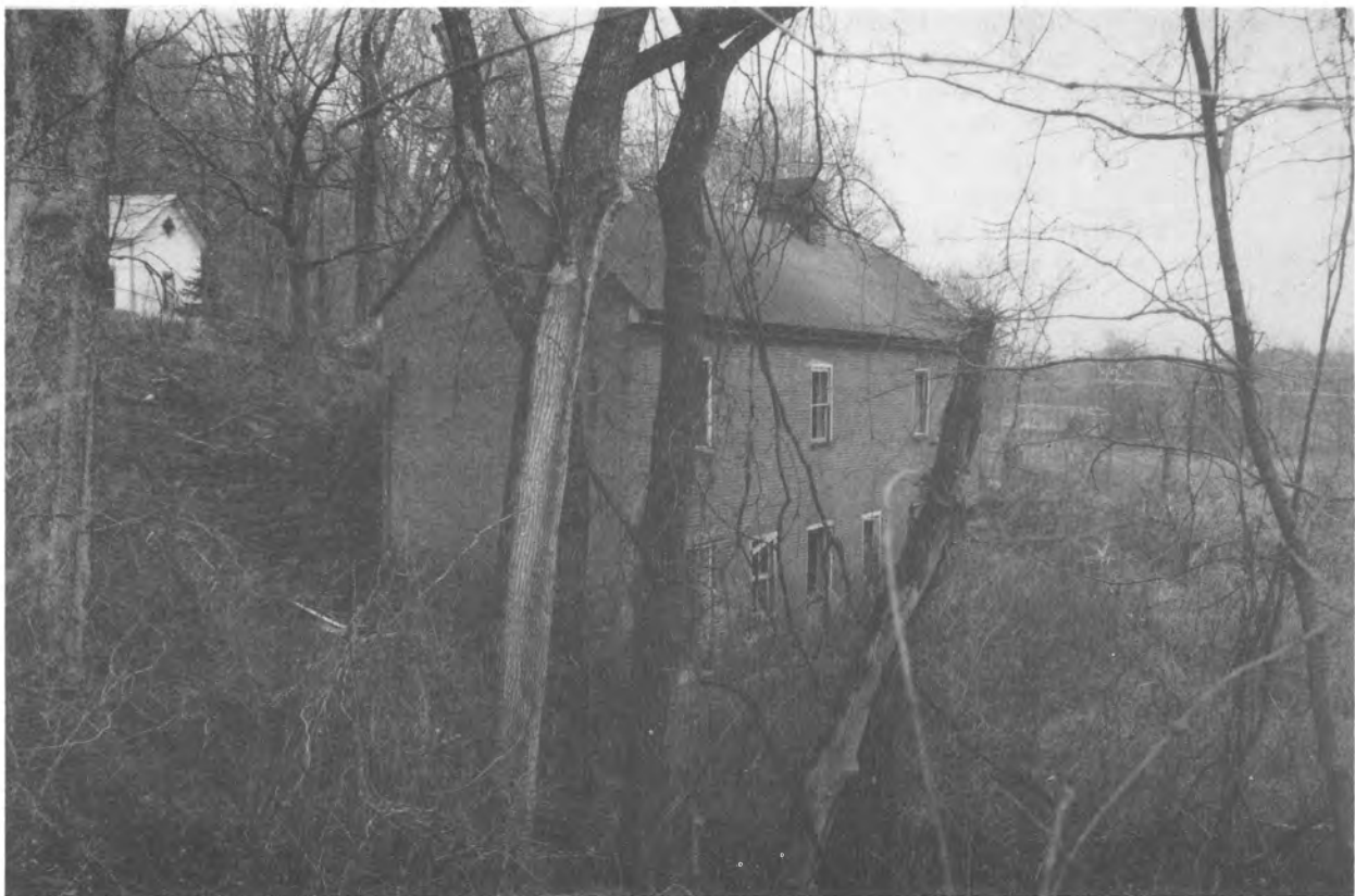
Figure 34. Cumberland Furnace Company Store (Dickson County 328).
