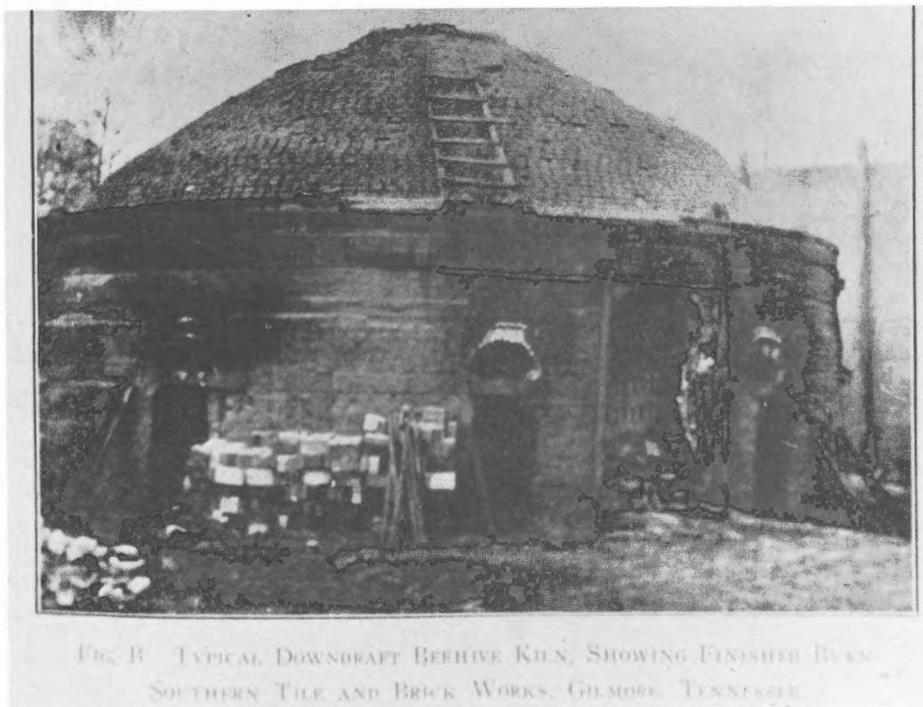
Figure 21. Example of downdraft kiln, late nineteenth to early twentieth-century type commonly used in West Tennessee for firing pottery as well as brick and tile (from Nelson 1911: Plate 5).
