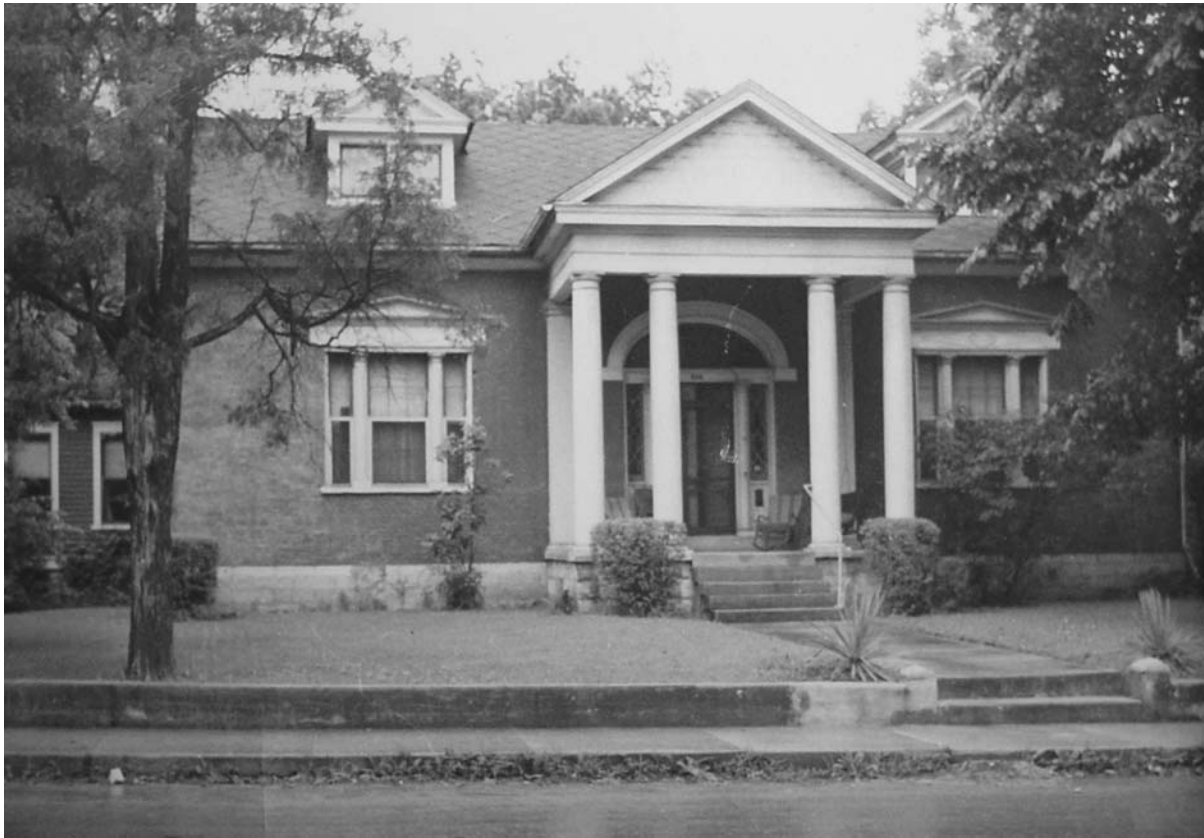
Figure 15. Photograph labeled “The Carter House circa 1940” (collections of the Carter House, Franklin, Tennessee).
