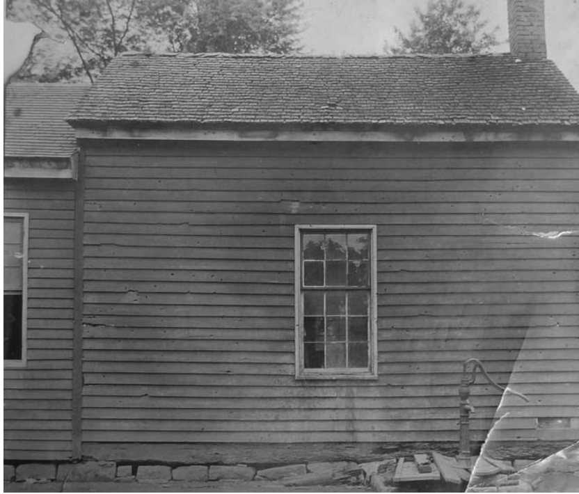
Figure 19. Ca. 1909 photograph of the “office” at the end of the west wing showing bullet holes in what during the Civil War was its south side (collections of the Carter House, Franklin, Tennessee; original came from Dr. Rosalie Carter).
