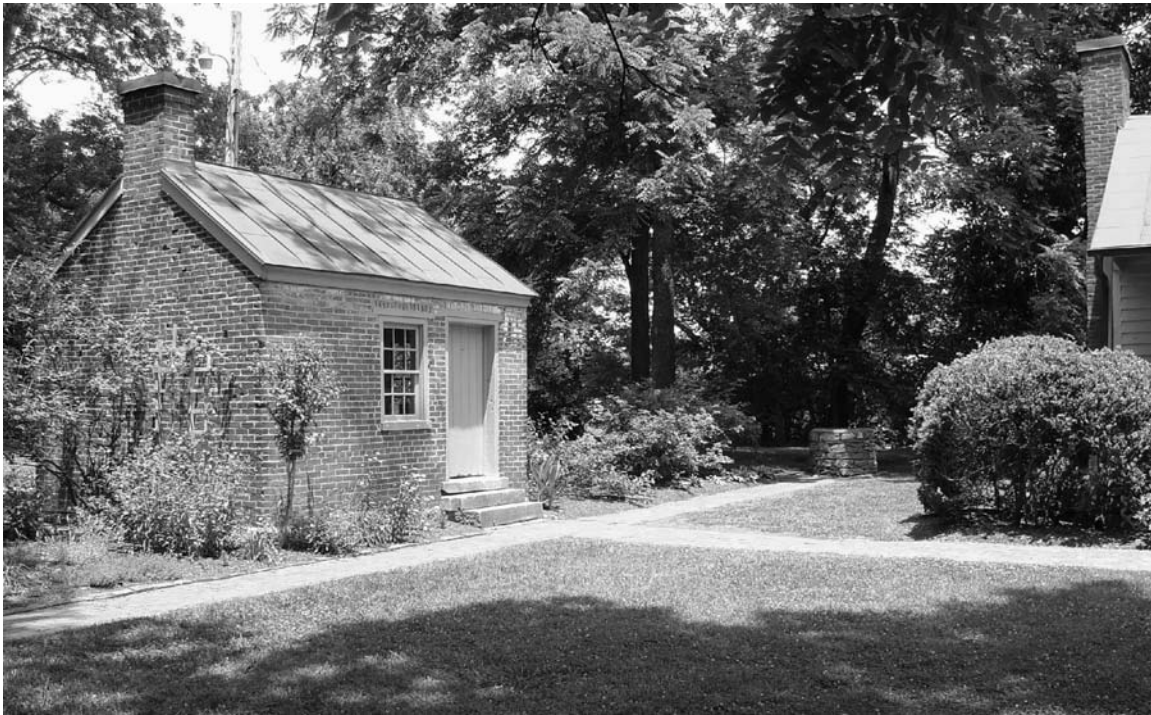
Figure 43. Carter House backyard area (facing northwest) showing sections of sidewalk between the back of the Carter House and the Kitchen.
