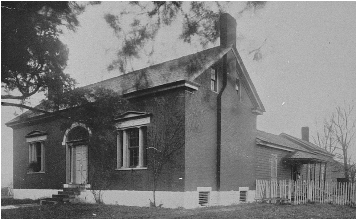
Figure 8. View of the Carter House facing southwest (from Scofield 1909:23).
