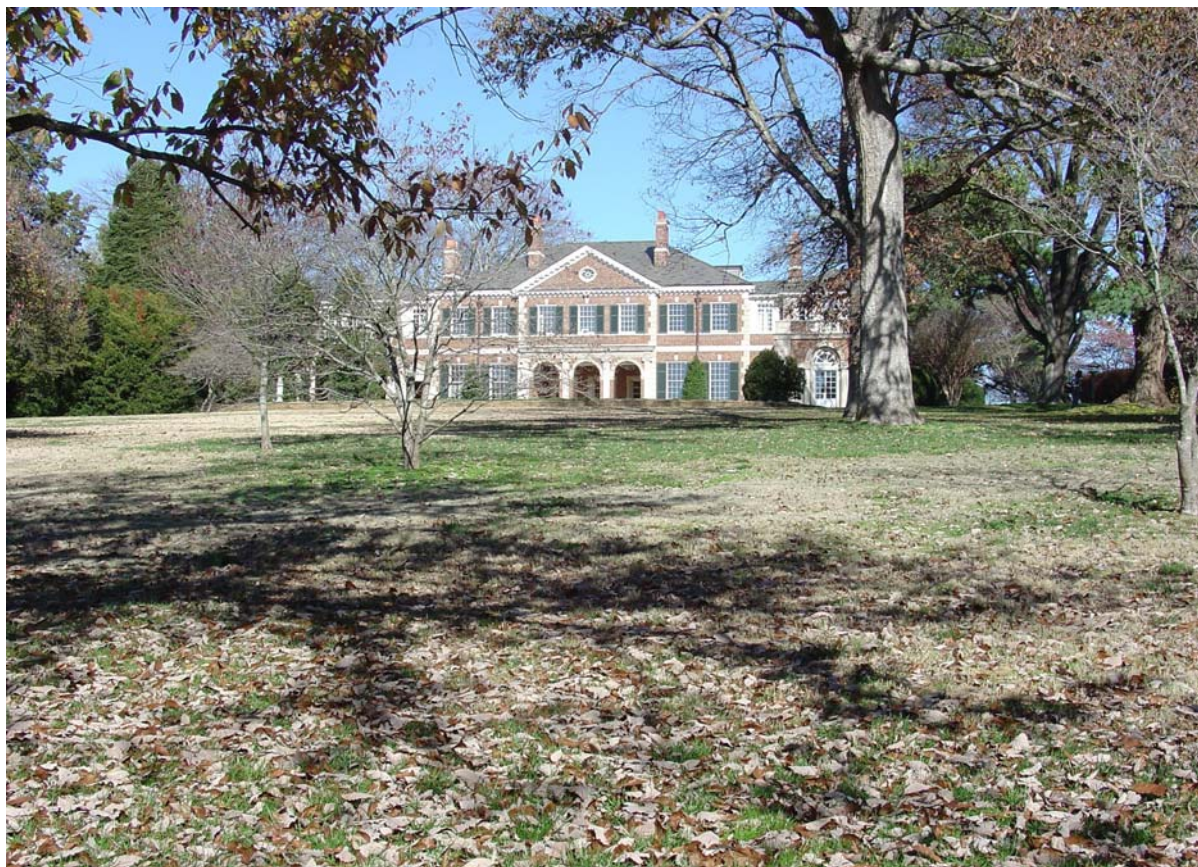
Figure 1D. View of the south (rear) side of the Executive Residence and its south terrace and sloping back lawn before the start of earth moving in connection with the construction of "Conservation Hall."
