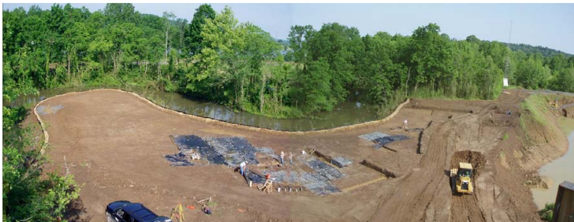
FIGURE 2. View of excavations at 40CH195, facing south.
