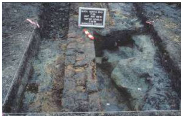
FIGURE 15. Portion of Feature 38 Foundation.
