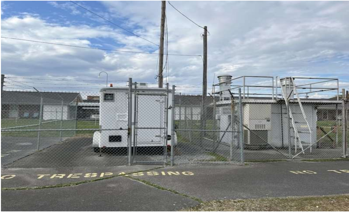
Photo: 009 Date: 03/05/26 Photographer: JMS Description: Site
