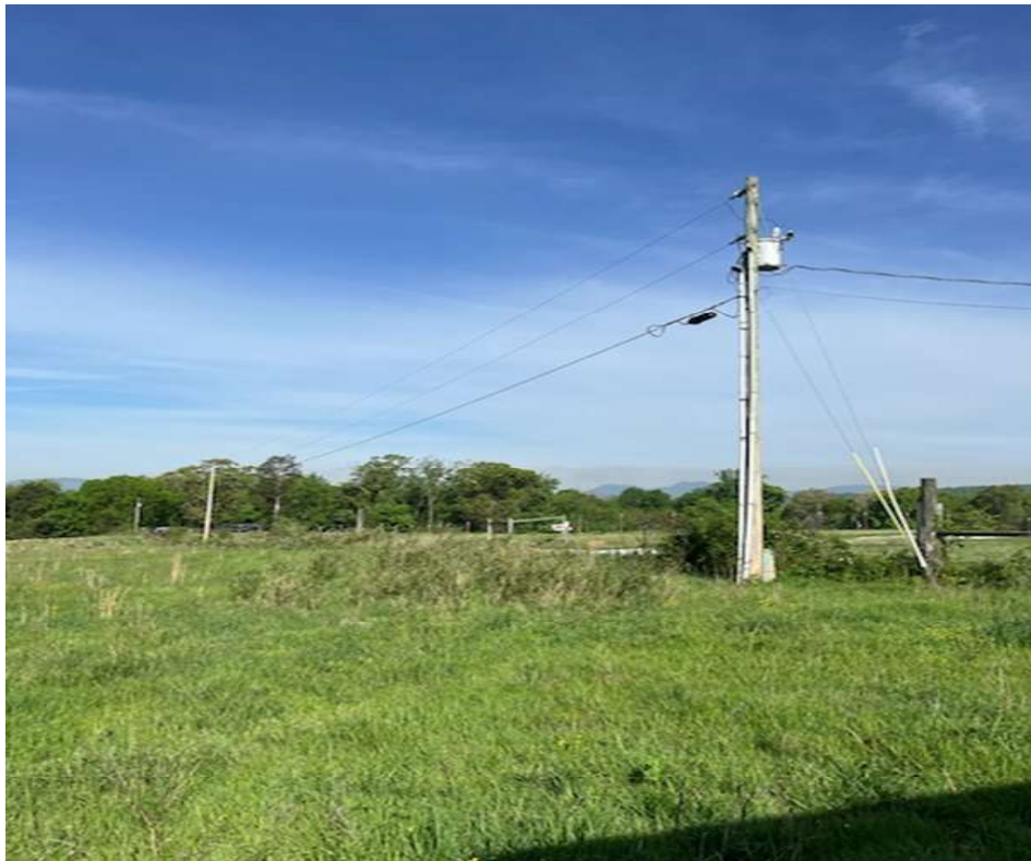
Photo: 008 Date: 04/15/26 Photographer: EMH Description: Northwest Directional
