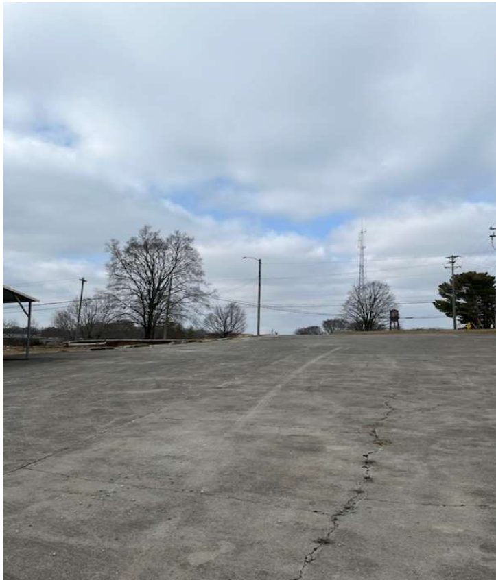
Photo: 008 Date: 02/05/26 Photographer: EMH Description: Northwest Directional
