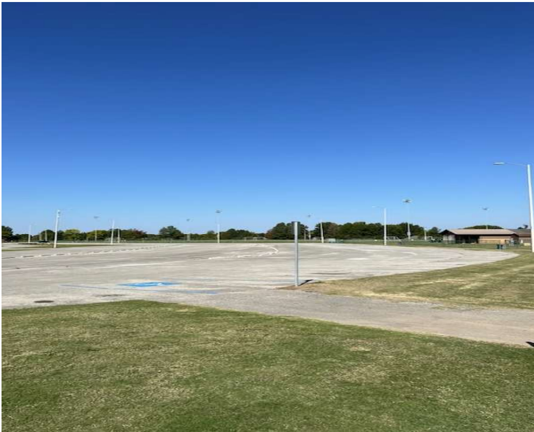
Photo: 008 Date: 10/16/25 Photographer: EMH Description: Northwest Directional
