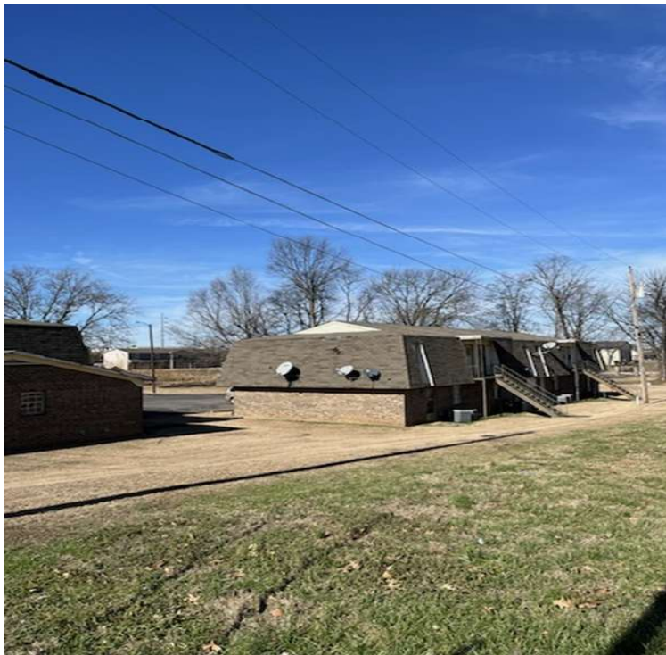
Photo: 008 Date: 01/13/26 Photographer: EMH Description: Northwest Directional
