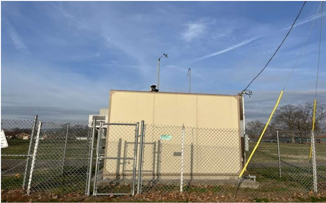
Photo: 009 Date: 03/06/26 Photographer: JMS Description: Site
