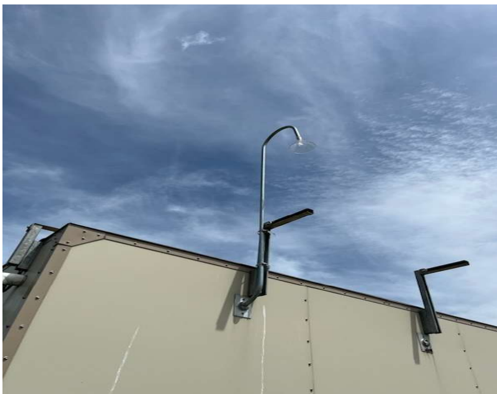
Photo: 010 Date: 04/14/26 Photographer: EMH Description: Probe
