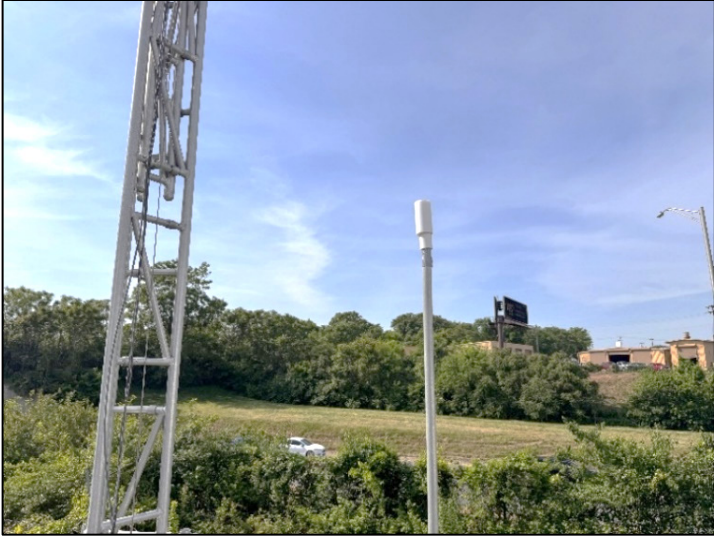
FIGURE 3-8: "NRS" – SOUTH VIEW
