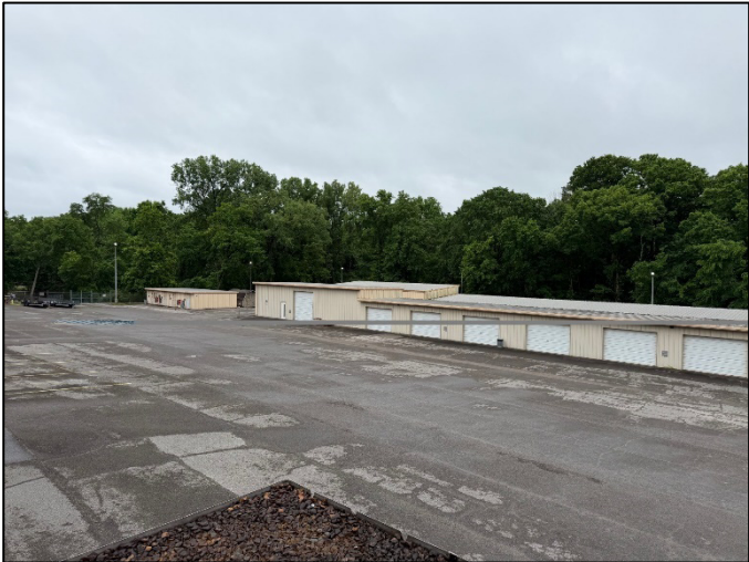
FIGURE 3-16: "PPD" – SOUTH VIEW
