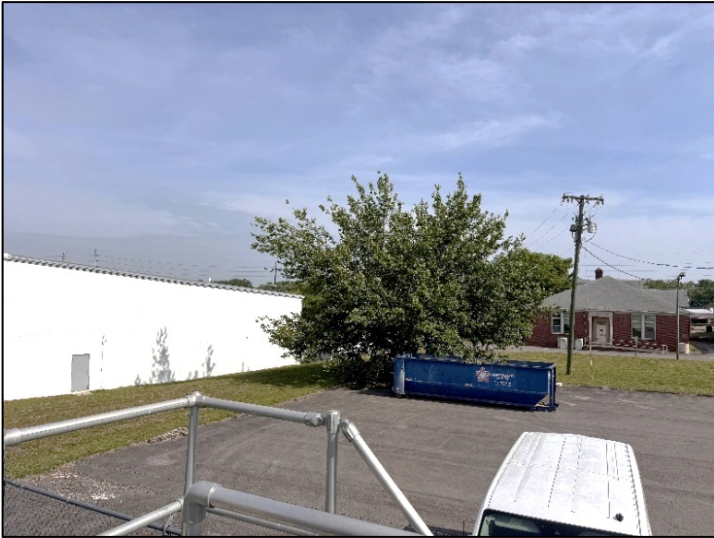
FIGURE 3-5: "NRS" – NORTH VIEW
