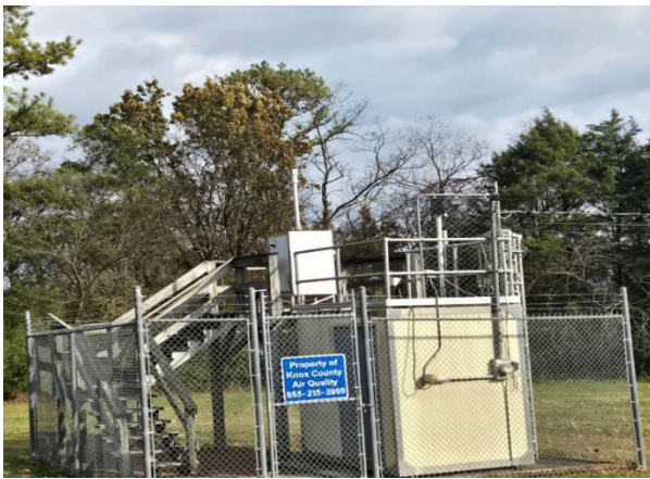
Figure 3.27 Springhill Site View
