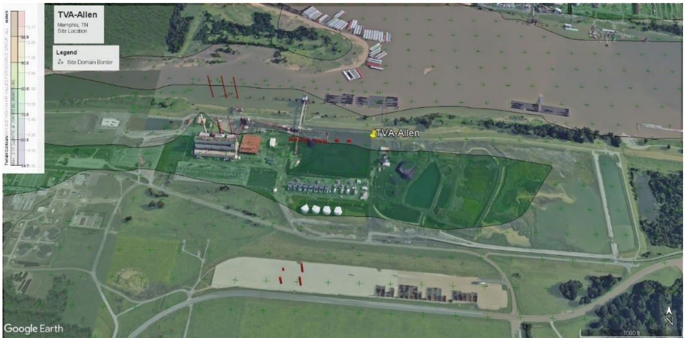
Figure 1: TVA-Allen site location
