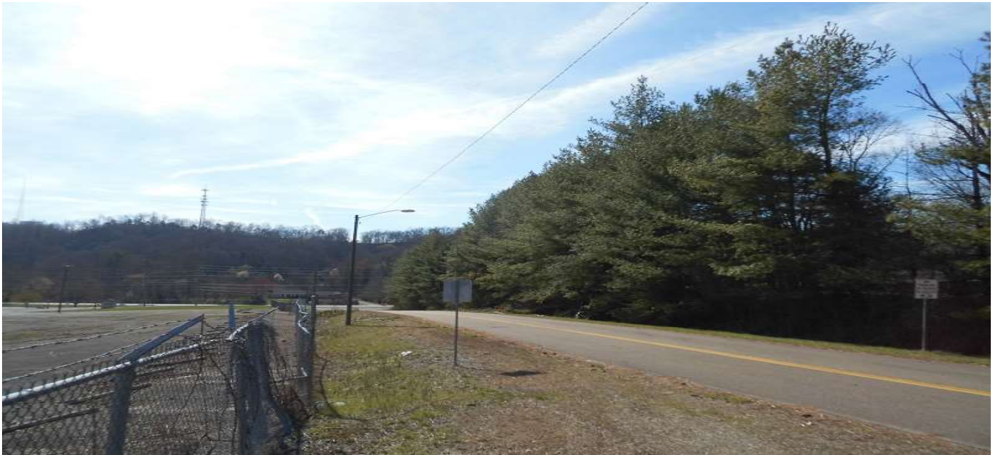
Photo: 005 Date: 03/16/23 Time: 11:15 am Photographer: EMH Description: South Diectional
