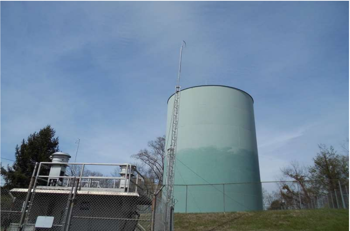
Photo: 010 Date: 03/16/23 Time: 1:30 pm Photographer: EMH Description: Tower
