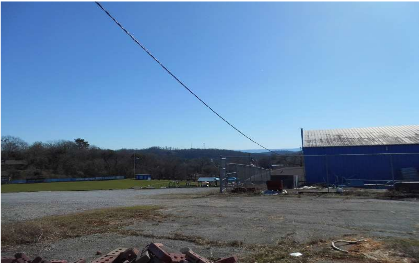
Photo: 004 Date: 02/06/23 Time: 12:35 pm Photographer: EMH Description: Southeast Directional
