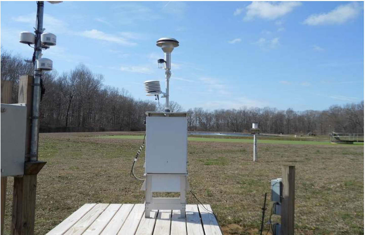
Photo: 010 Date: 02/23/23 Time: 11:10 am Photographer: EMH Description: Monitor
