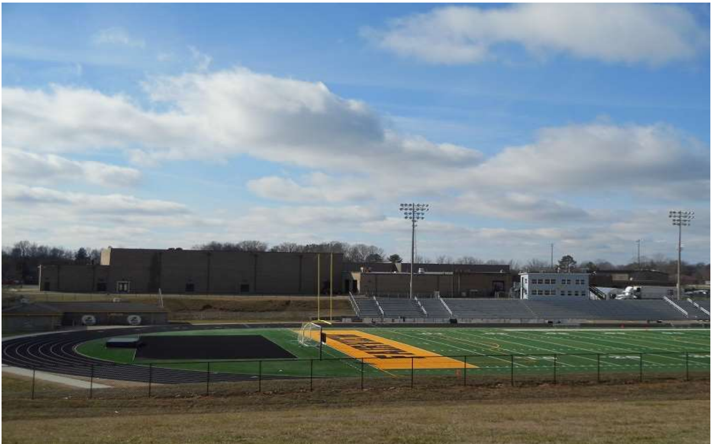
Photo: 006 Date: 01/20/23 Time: 10:45 am Photographer: EMH Description: Southwest directional
