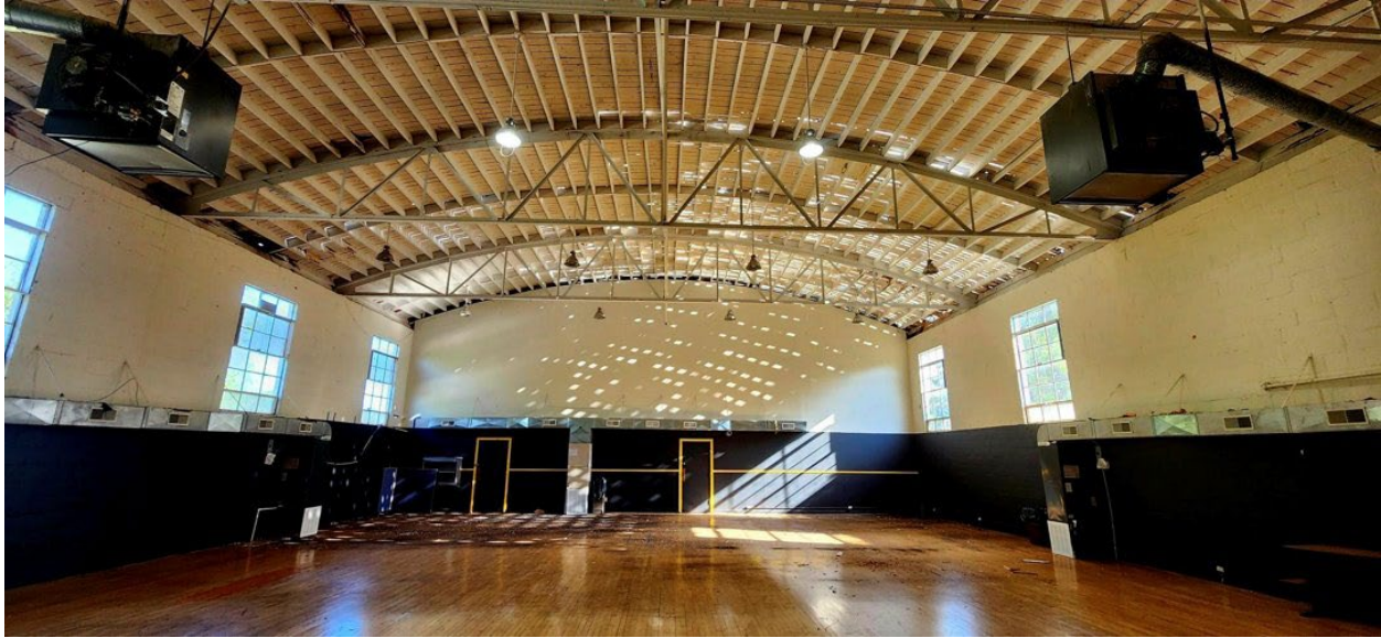
Photo 7: A New Roof in a Connected Community Facility in Franklin County, Tennessee
