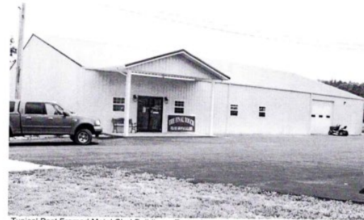
Typical Post Framed Metal Clad Building – Example
