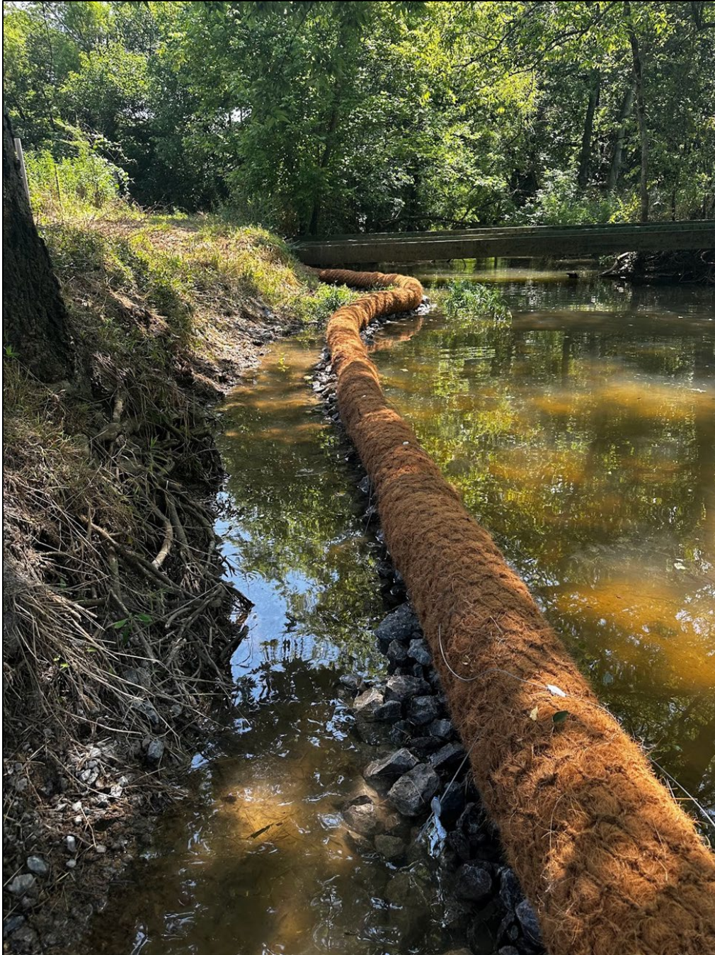
Photograph 2: Streambank stabilization along Lytle Creek
