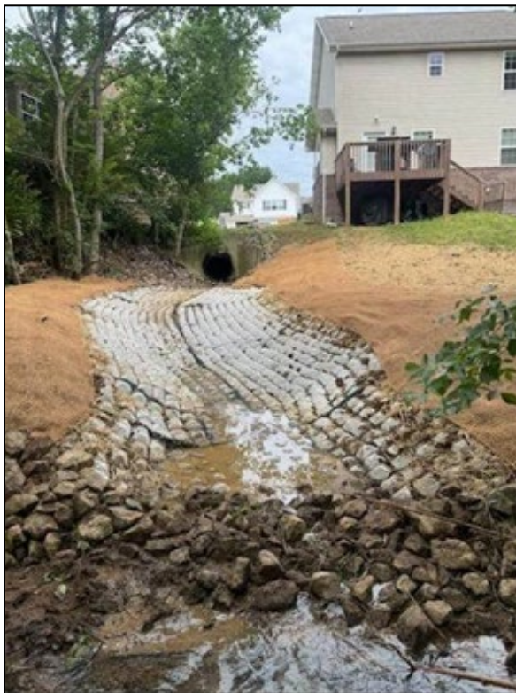
Photograph 1: Renovation of stormwater outlet
