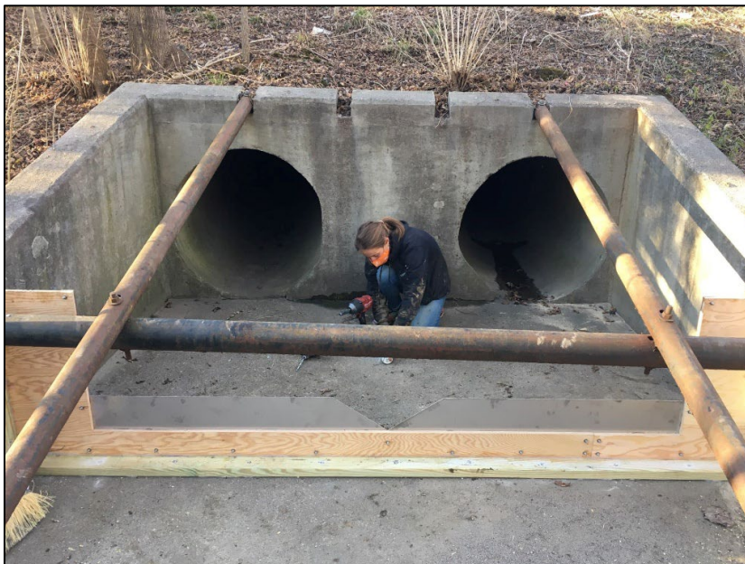
Photograph 1: UT graduate student installing monitoring equipment
