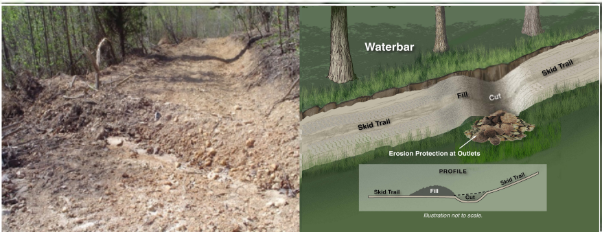
Figure 7a. Water bar construction
