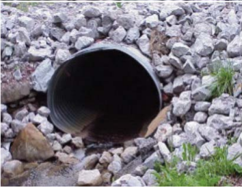
Figure 9. Riprap to stabilize outlet
