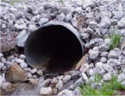
Figure 9. Riprap to stabilize outlet
