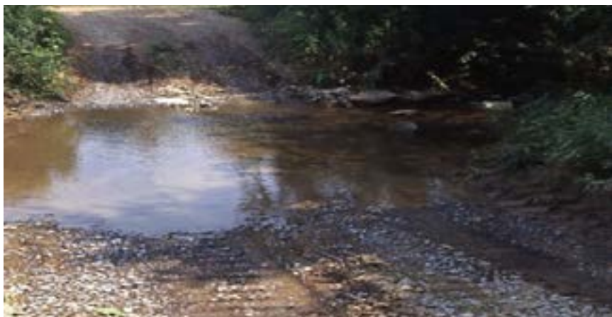
Figure 8b. Correctly Constructed Ford
