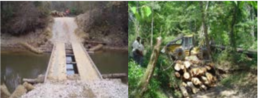
Figure 10. (left) Portable steel bridge suitable for hauling. (right) Temporary pole bridge suitable for skidding and hauling. Temporary bridge structures should be removed after use.
