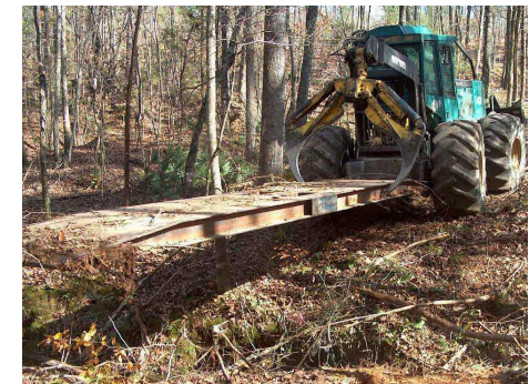
Steel skidder bridge being installed with grapple skidder
