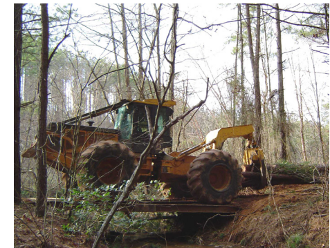
Steel skidder bridge supporting skidder over drainage
