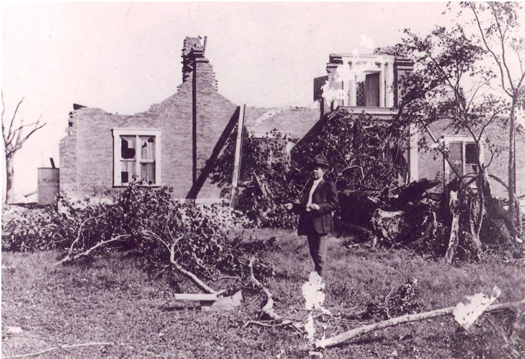
Figure 2. Post tornado photo of house, side elevation.
