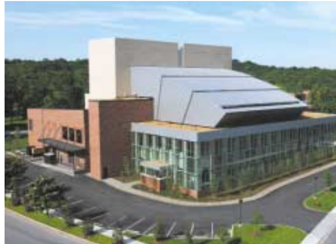
SSRCx provided commissioning services for mechanical, plumbing, fire protection and electrical systems for Vanderbilt University's Blair School of Music, a state-of-the-art musical instruction facility. Return on investment for this project resulted in $7 for every $1 spent.
