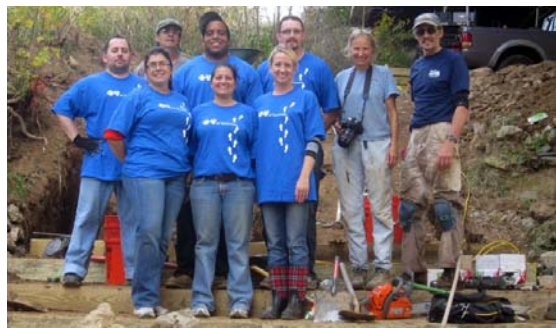
TN State Parks thanks all its partners for their volunteer work in completing another public river access site along the popular Harpeth River State Park Blueway in Cheatham County. More than 360 hours of labor from 57 volunteers completed this project in just seven days - with the final push to completion on Fri., Nov. 11.
