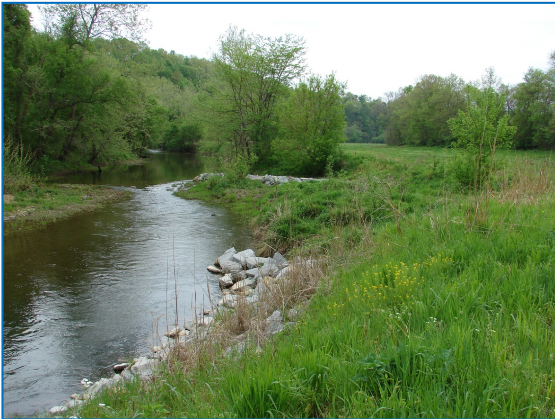
Stream bank restoration
